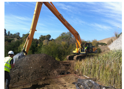
Top of slope repair
