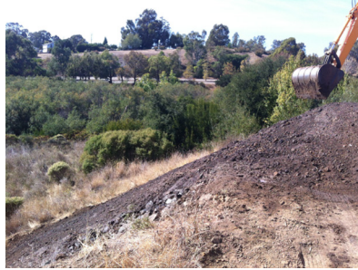
Top of slope repair
