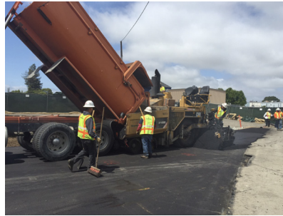
Asphalt delivery and placement
