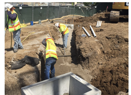
Placement of storm drain system
