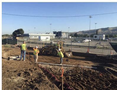
Excavation of roadway
