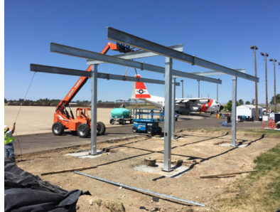
Canopy structural steel erection
