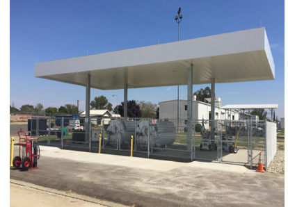
Final LOX station construction
