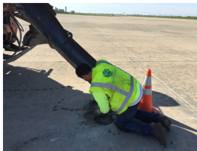
Tie down concrete placement (1 of 108)
