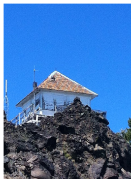
Condition prior to project start
