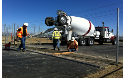
Main gate construction
