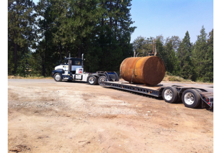
Tank ready for transport to disposal facility
