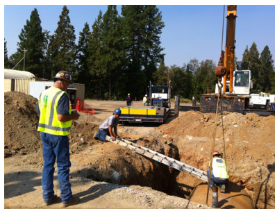
Rigging of the tank
