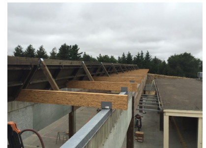
Completed baffle construction
