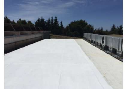
Armored steel roof
