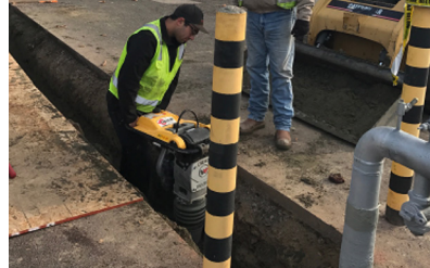
Pipe bedding compaction
