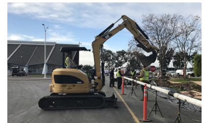
Pipe lifting into trench
