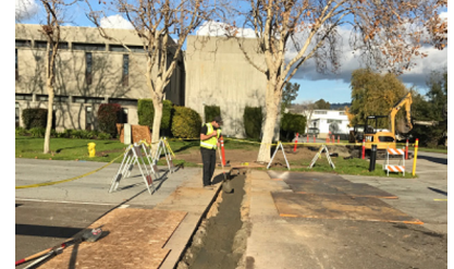
Controlled density fill placement
