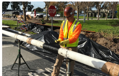
Pipe slice corrosion wrapping
