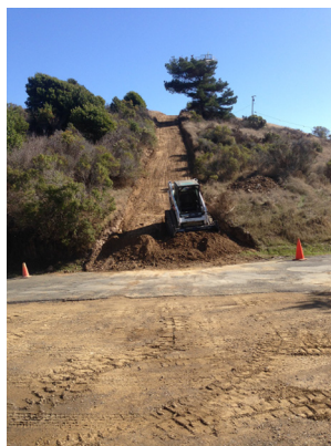
Access road repairs
