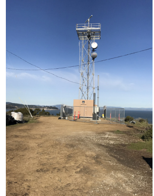
Final project installation
