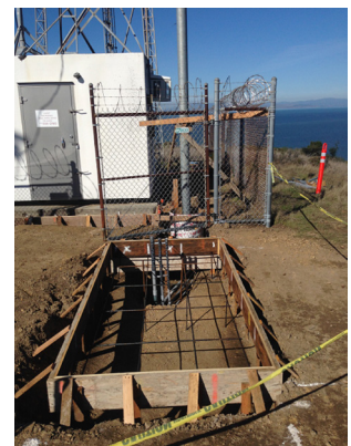
Concrete formwork
