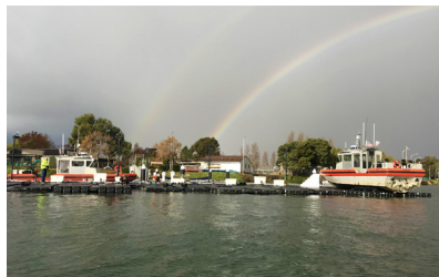
Jet dock work underway
