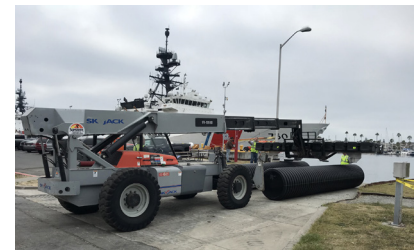
Rebuilding of new jet docks
