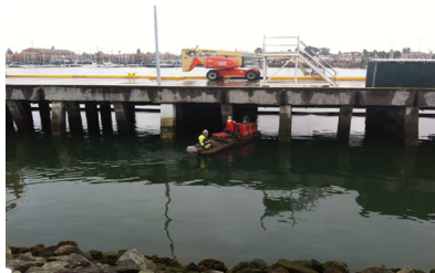
Replacement of under pier sewer system
