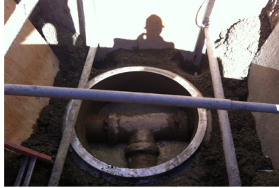
Placement of new manhole invert
