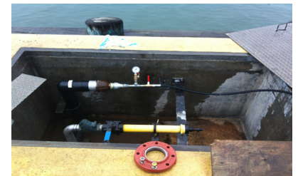
Successful air test of new pier sewer system
