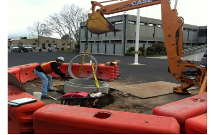
Placement of top manhole section
