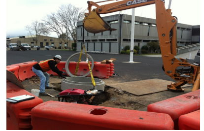
Placement of top manhole section
