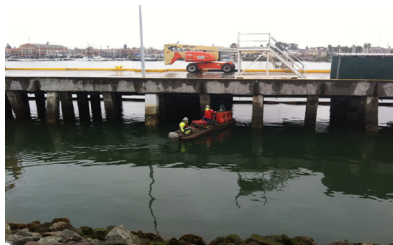
Replacement of under pier sewer system
