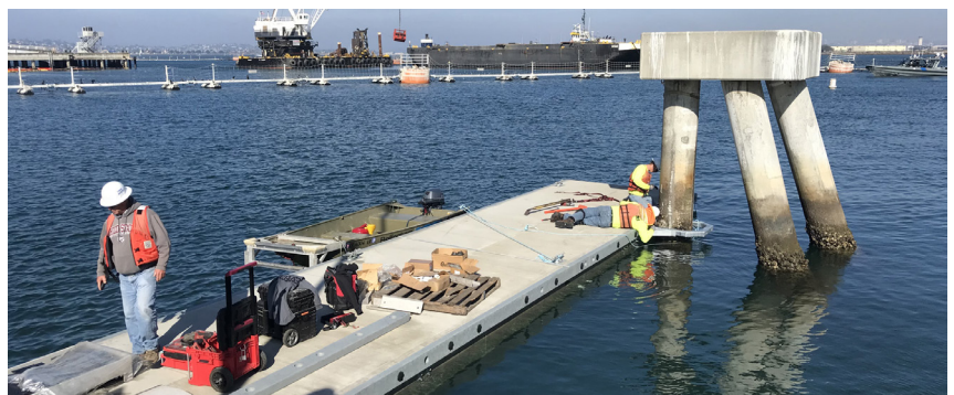
Installation of new dock
