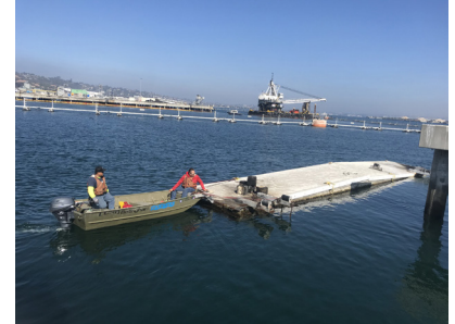
Removal of existing dock
