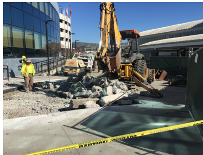
Existing concrete removal
