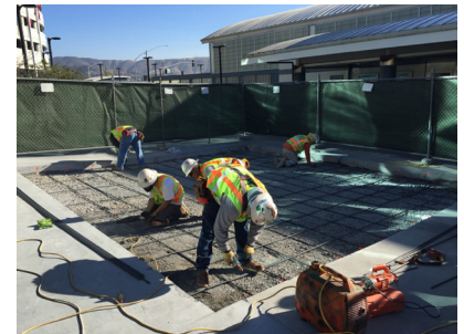
Concrete reinforcement placement
