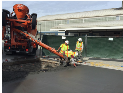
Concrete placement
