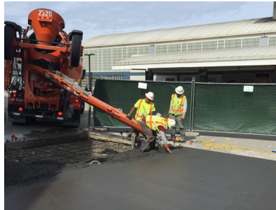
Concrete placement
