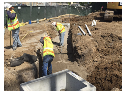
Placement of storm drain system
