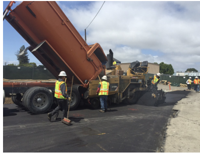
Asphalt delivery and placement
