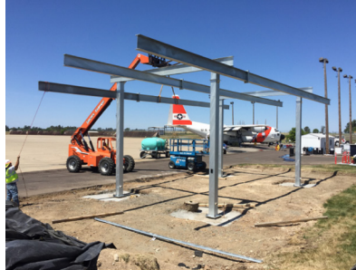
Canopy structural steel erection
