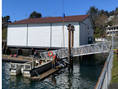
New pile guide assembly installation
