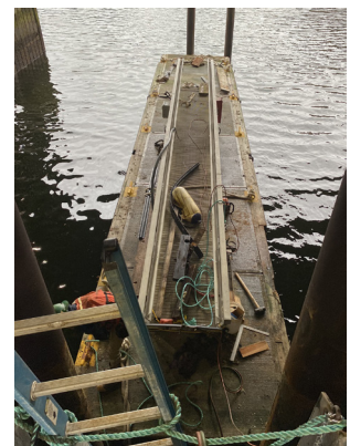
Existing floating dock condition
