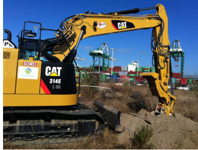
Test pit excavation
