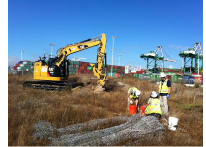
Testing of excavated material
