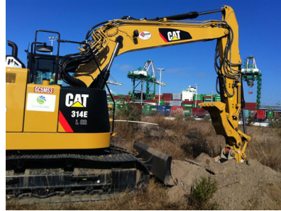
Test pit excavation
