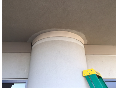
Birdslide final installation
