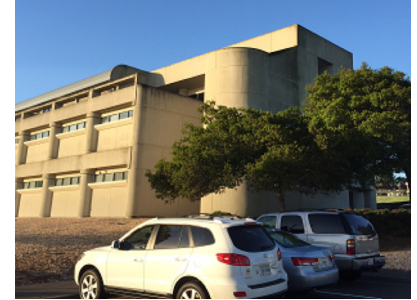
Bauer Building post birdslide installation
