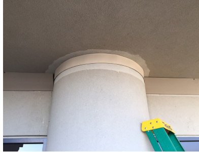
Birdslide final installation
