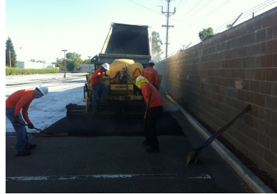
Paving operations in parking lot
