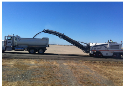
Removal of existing asphalt
