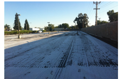
Placement of geomembrane
