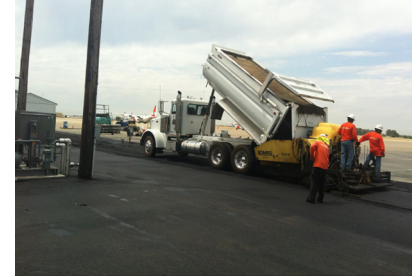
Paving operations near TARMAC
