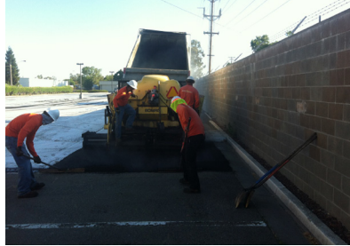
Paving operations in parking lot
