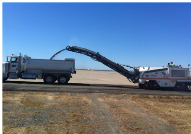
Removal of existing asphalt
