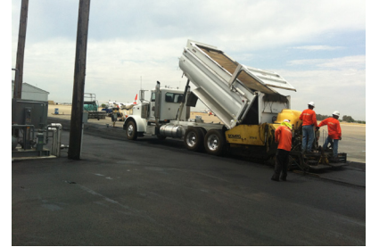
Paving operations near TARMAC
