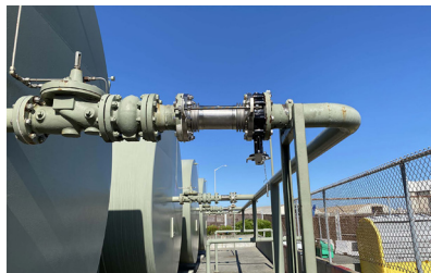
New flex bellow coupling with valve
