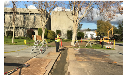
Controlled density fill placement
