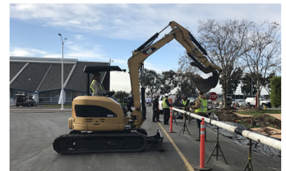
Pipe lifting into trench
