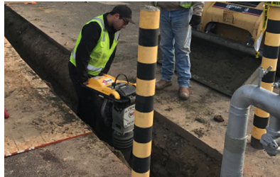
Pipe bedding compaction
