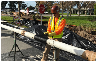
Pipe slice corrosion wrapping
