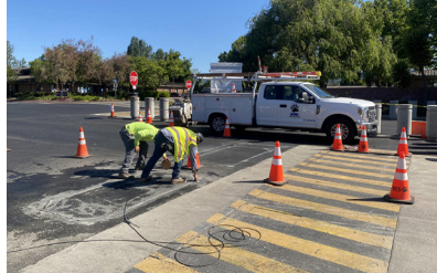
Ground loop installation
