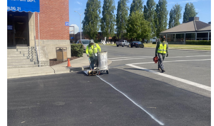
Thermoplastic restriping
