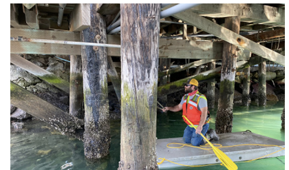
Installation of conduits under pier
