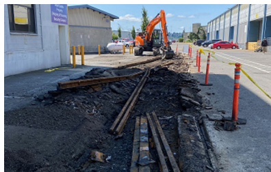
Railroad track removal
