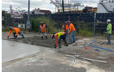
Concrete placement over sinkhole area
