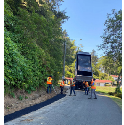
Paving of Trench
