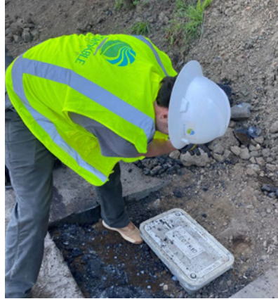
Lighting Circuit Vault Installation
