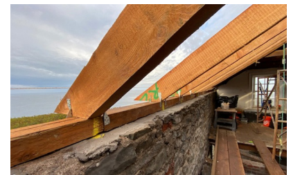
Roof framing repairs
