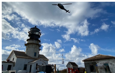
Air operations and delivery of materials
