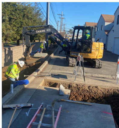
Trenching for new electrical cable
