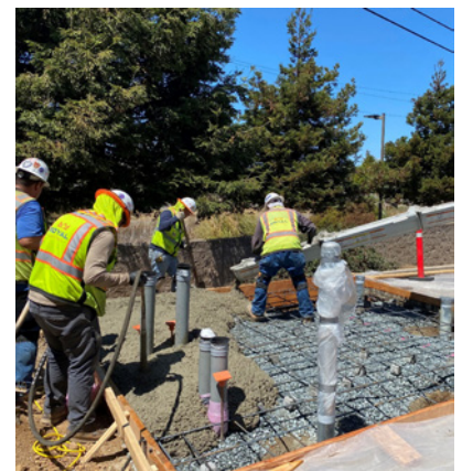
New switchgear pad construction
