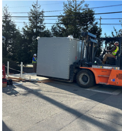
Placement of new switchgear
