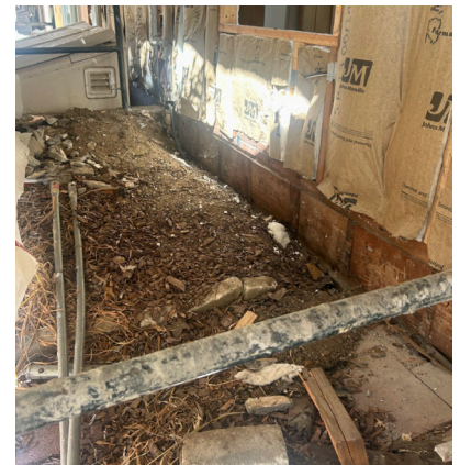
Exterior Sheathing Removal
