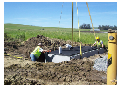
Filterra system placement
