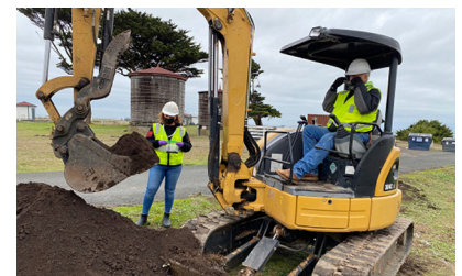
County PID testing of excavated soil
