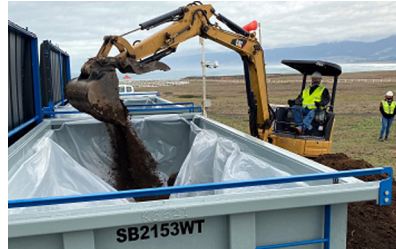
Placing of soil in lined bins
