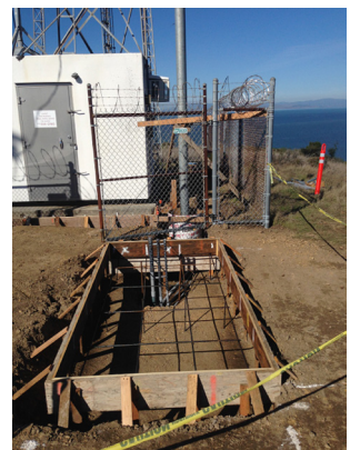
Concrete formwork
