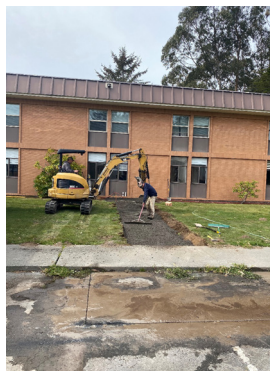
New front entry construction
