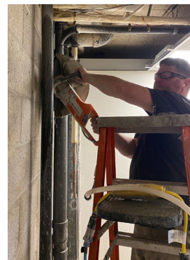
Saw cutting for new door opening
