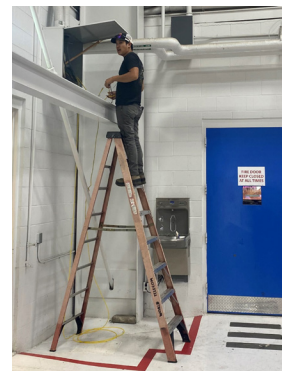
Installation of new fiber optic cable
