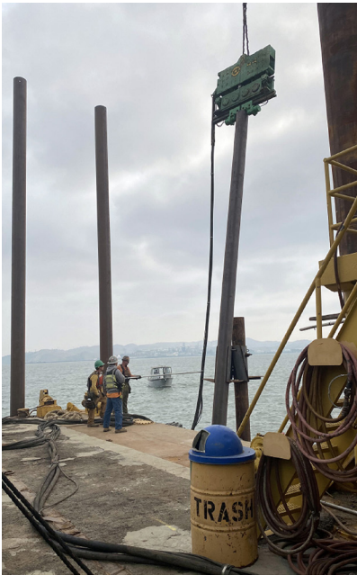
Vibratory pile driving for 3-pile structure
