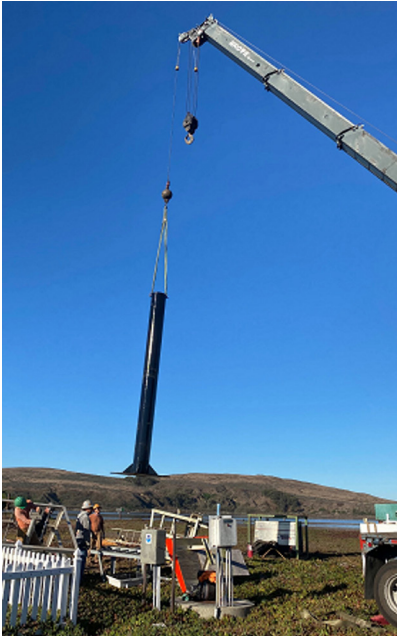
Construction of Bodega Bay Range C Rear Light
