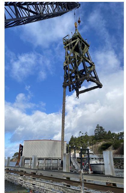
Light 13 structure removal
