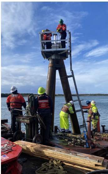
Light 13 ladder/light installation
