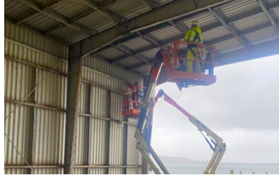
Interior bird netting repairs
