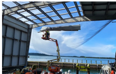
Removal of roof panels
