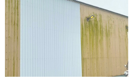
Siding panel replacement complete
