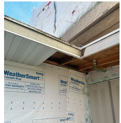
New Soffit and Building Wrap
