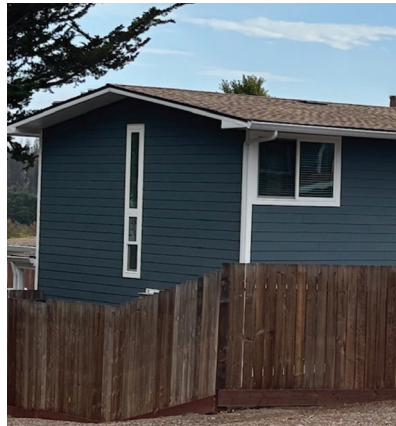
New Siding, Windows and Asphalt Roof
