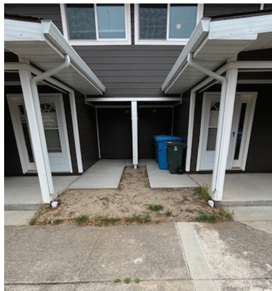
New Exterior Siding, Doors, Windows, Gutters, Downspouts and Concrete
