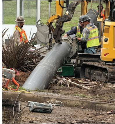
Storm Drain Repairs
