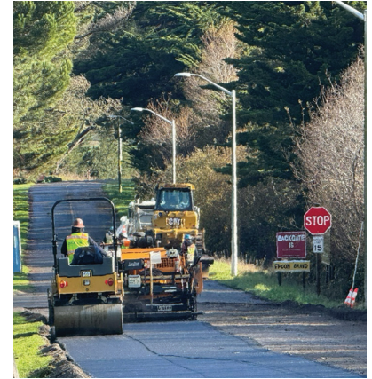
Asphalt Paving in Progress
