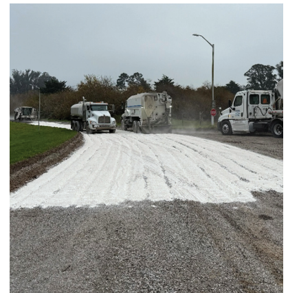
Lime Stabilization Application
