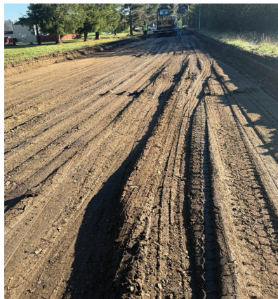
Pavement Removal and Subbase Preparation
