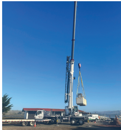
Gasoline Tank Removal
