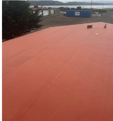
New TPO Roofing
