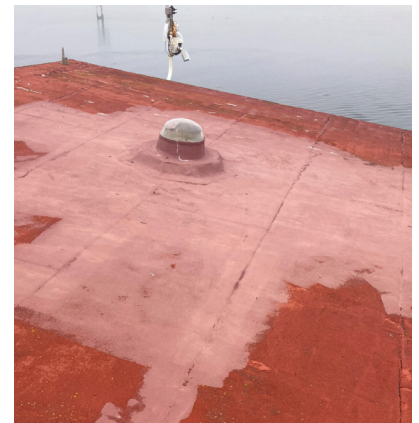
Prior Roofing Condition
