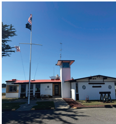
Administration Building at Project Completion
