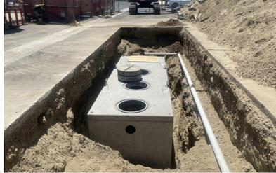
New tank and temporary by-pass line installed
