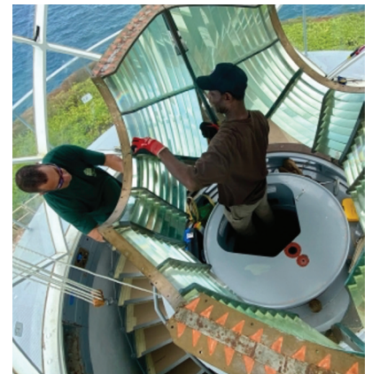
Fresnel Lens Disassembly
