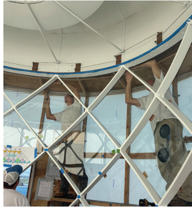
Glazing Panel Installation
