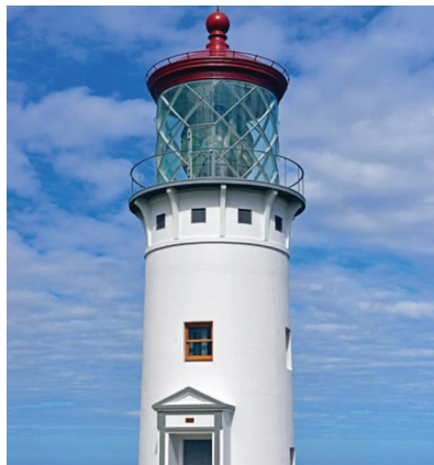
Kilauea Point Lighthouse Project Complete
