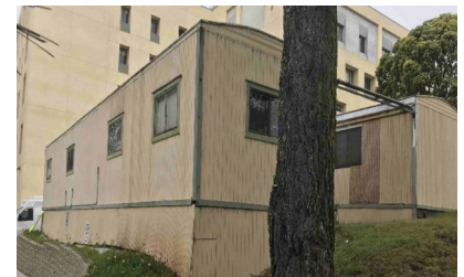
Trailer T-28 with adjacent retaining wall
