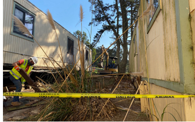
Removal of the exterior decks
