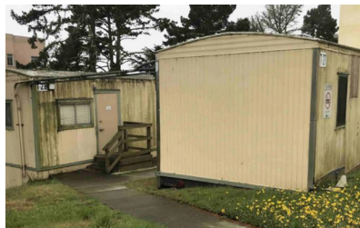
Existing trailers T-27 and T-28
