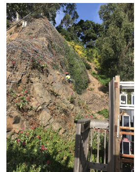
Draped mesh installation
