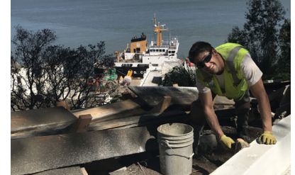
Upper spillway construction
