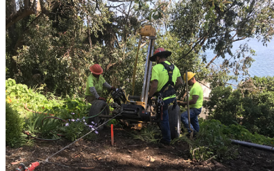
Draped mesh anchor installation
