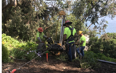
Draped mesh anchor installation
