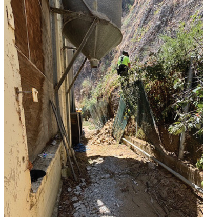
South Hillside Scaling of Loose Rock
