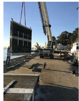
Installation of new panels
