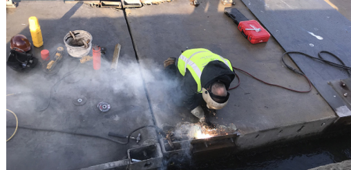
Floating dock repairs
